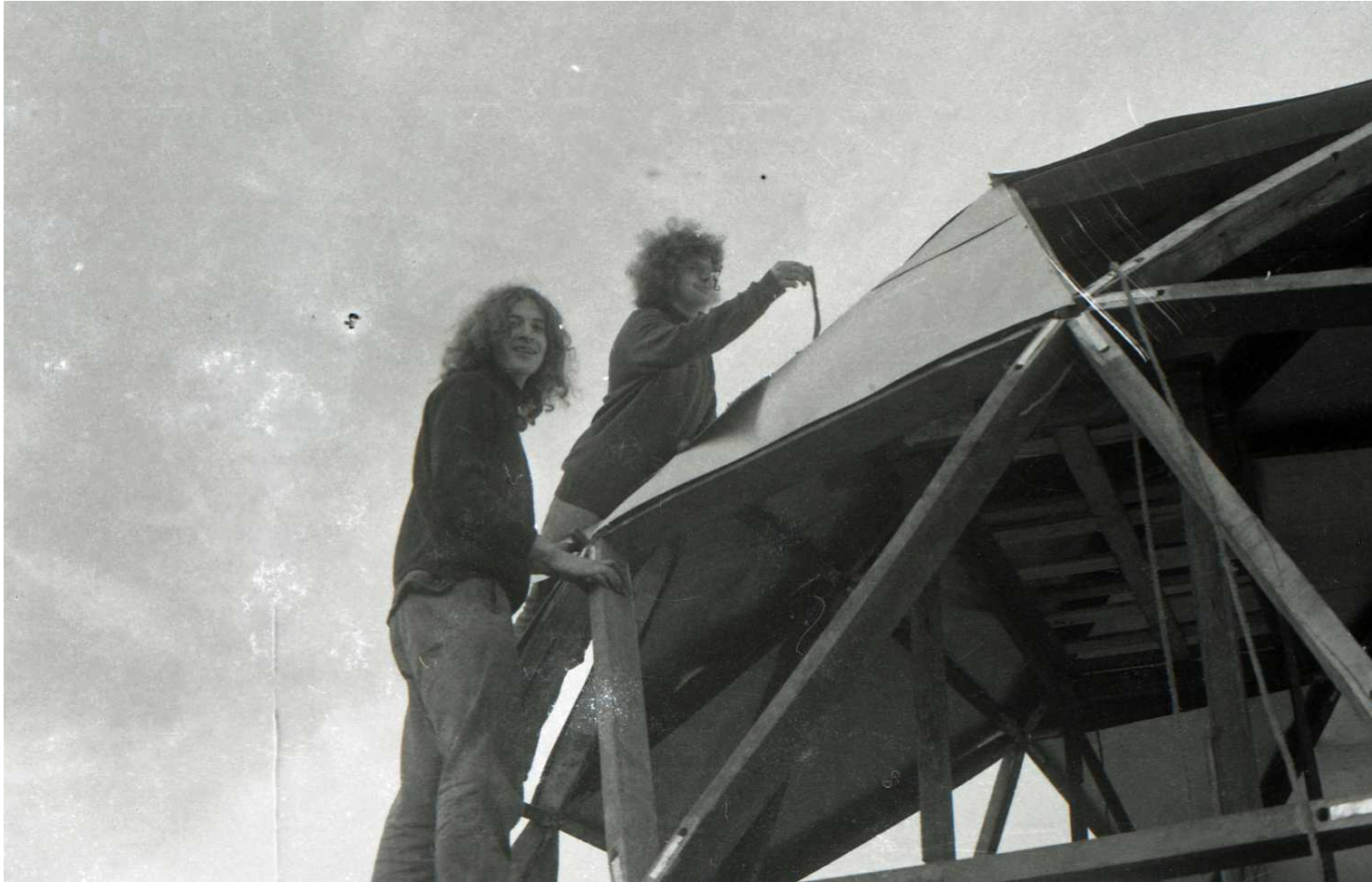
Paul and Lowen. Dome under construction.
