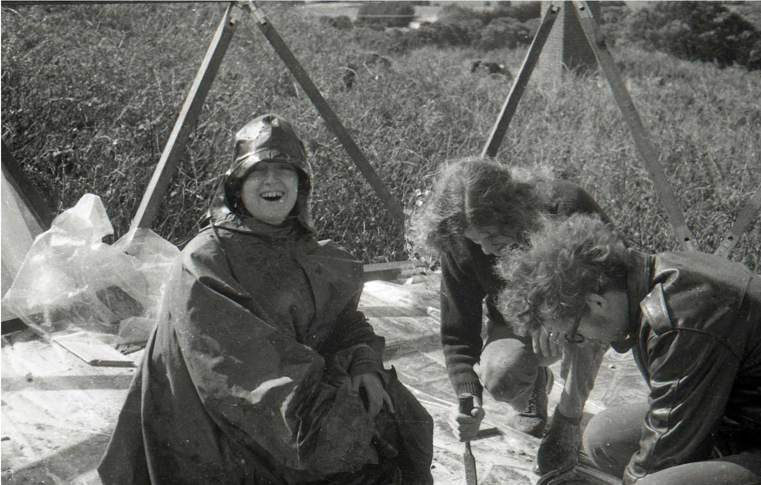
Morgan, Philip and Gerry. Dome under construction.
