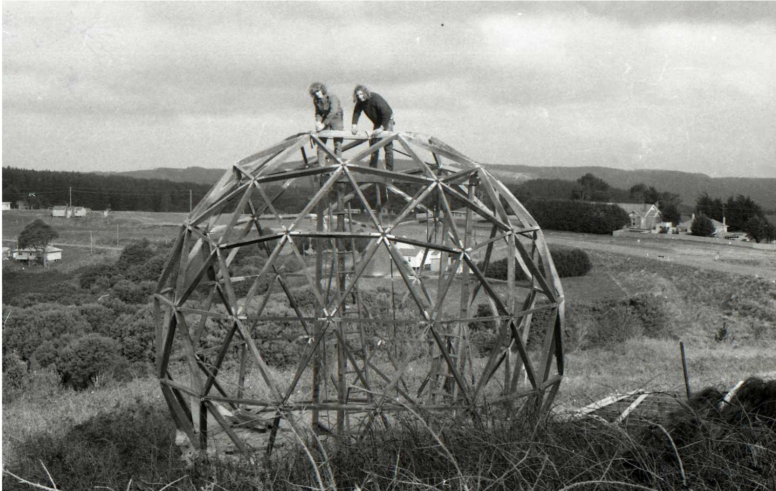
Philip and Paul. Dome under construction.
