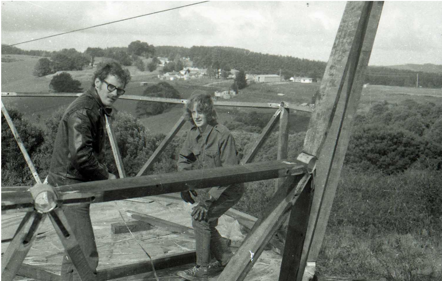
Gerry and Philip. Dome under construction.
