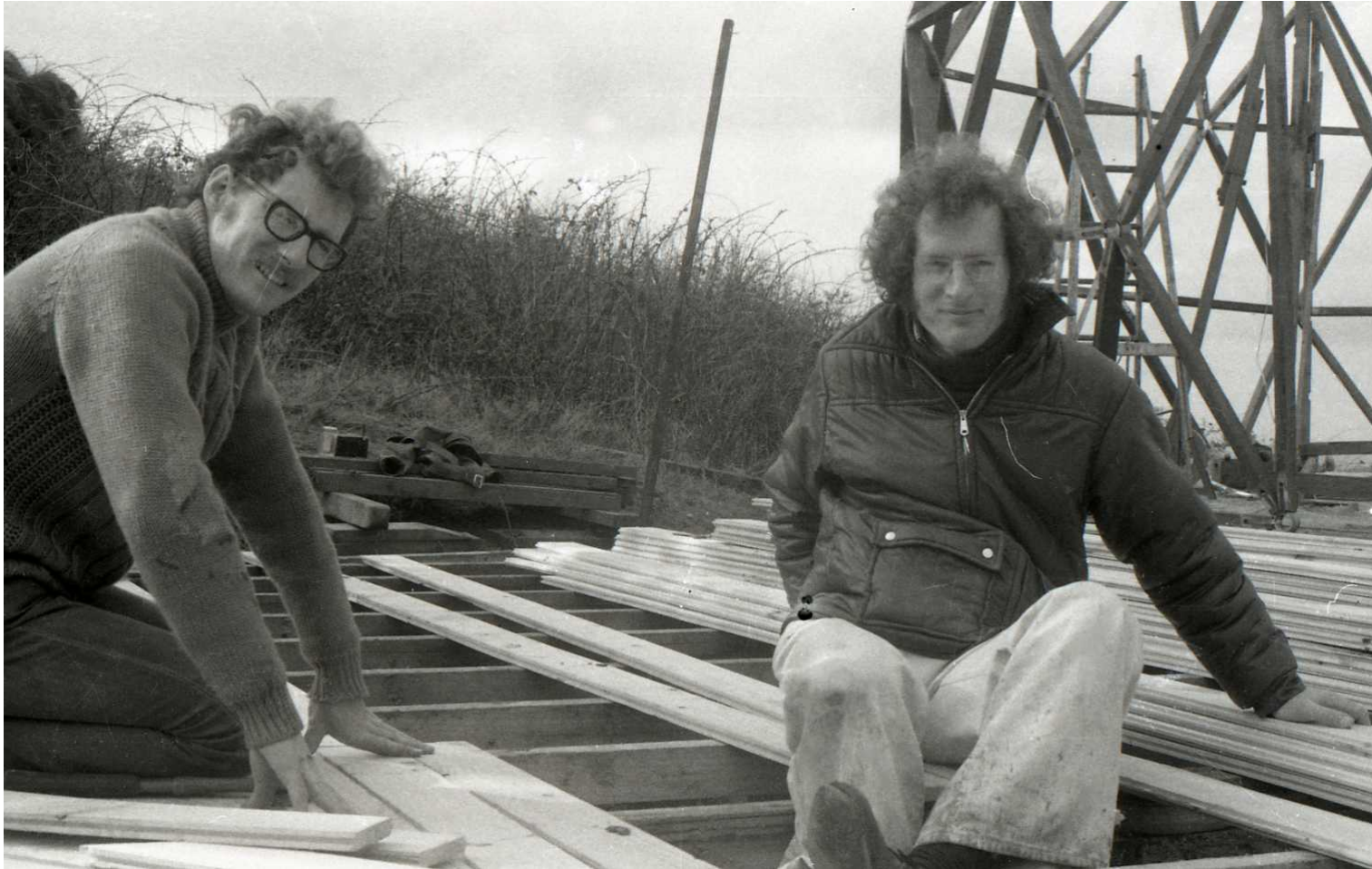
Gerry and Tony. Dome under construction.
