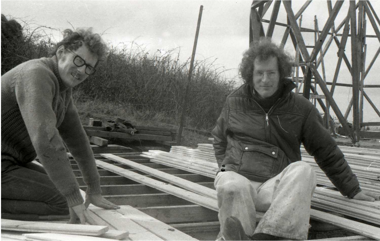
Gerry and Tony. Dome under construction.
